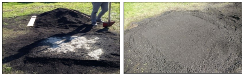
Figure 56 - Cement mixing and stabilized block (1.20x1.20x0.20 m)
