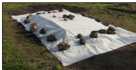
Figure 57 - Protection system to ensure an adequate curing
