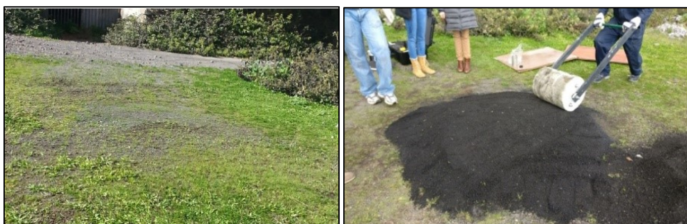
Figure 53 - Test area and manual roller compactor of the University of Catania
