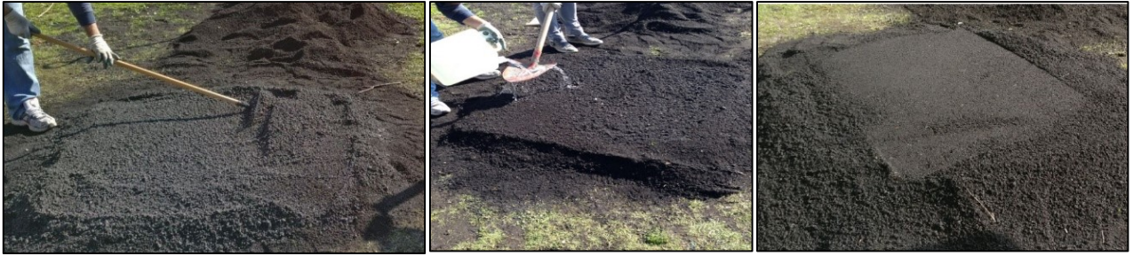
Figure 54 - Laying of the layers, hydration with water and compacted ash
